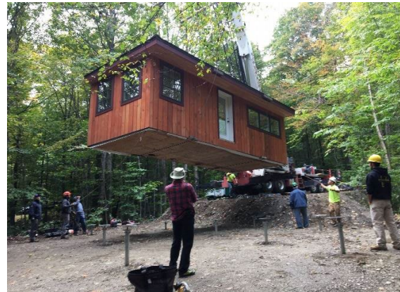
A portion of the Chittenden Brook Hut being lifted into place (opened fall 2018).
